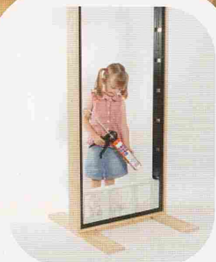
Line silicon across centre of frame and bed in 1st row of glass blocks
